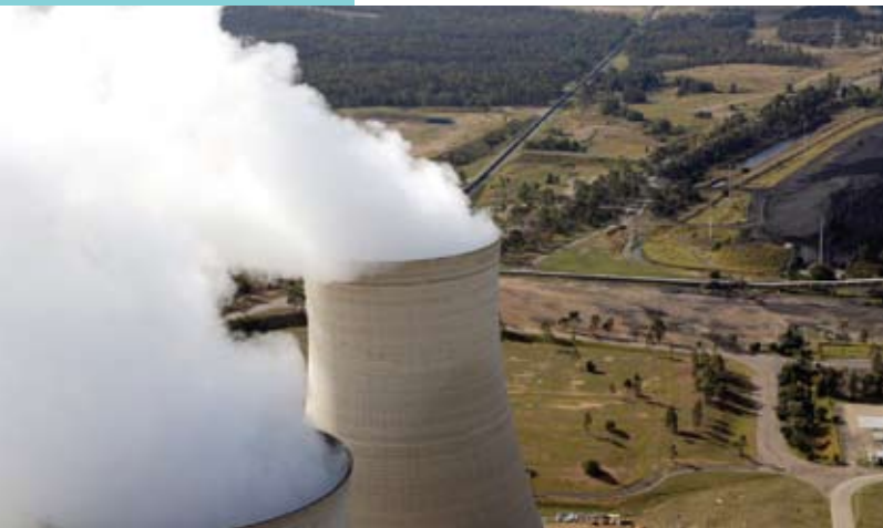
View of the conveyor from behind the Power Station.
